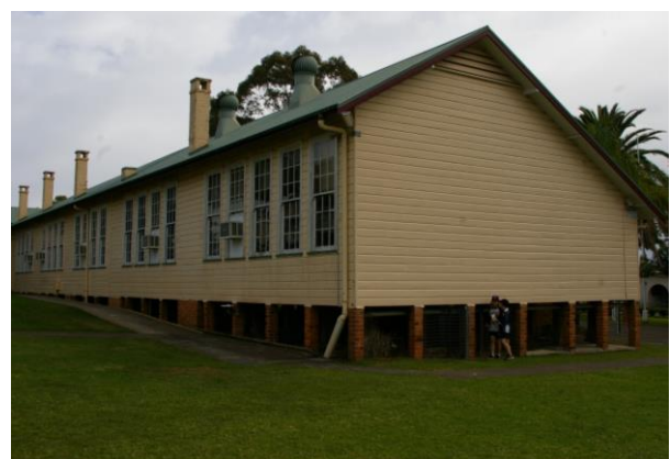
Figure 7: Typical arrangement of four double hung windows on the south facade of building 6 at Wauchope Public School. (Source: Conrad Gargett)
