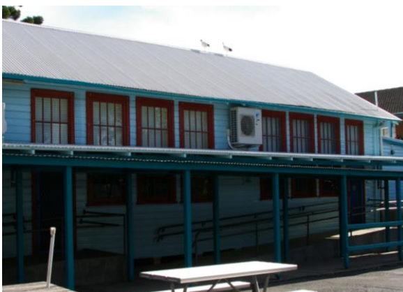
Figure 6: Typical arrangement of four double hung windows on the South-eastern facade of building B at Coffs Harbour Public School. (Source: Conrad Gargett)
